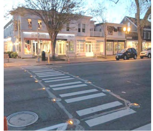
Lighted Crosswalk Example
